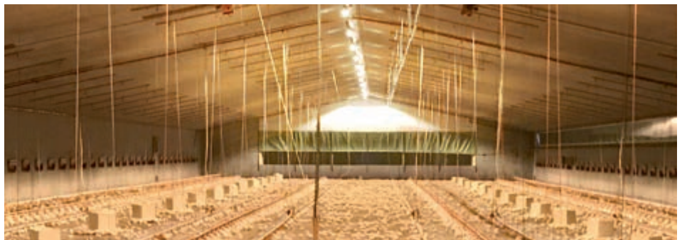
Aurora 540: an entire row of lamps can be saved in low houses due to the batwing optics
