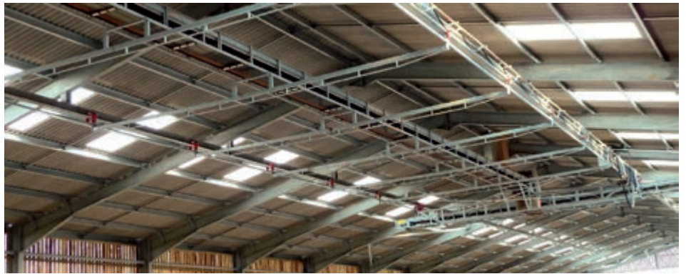
View of an H-shaped distributor
