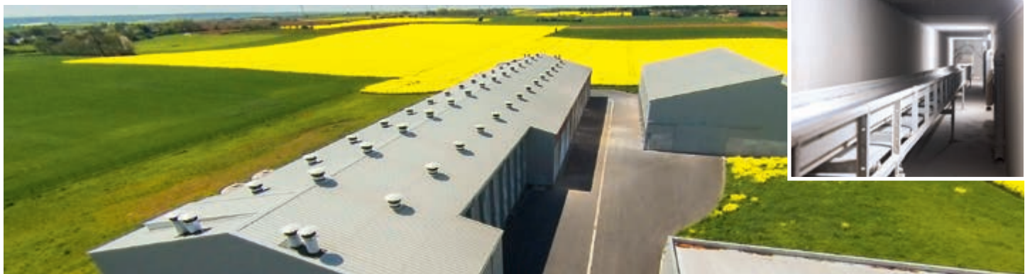
Environmentally-friendly solution: two OptiPlate dryers for 205,000 layers at the barn's long side; the dried manure is transported into the manure storehouse underground
