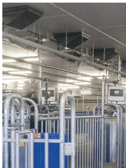
Fin heater as a full-space heating system – ideal in combination with ceiling inlets
