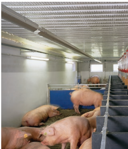
Delta pipe – ideal for installation below the DiffAir ceiling
