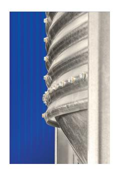
**CRIMP:** Crimp at room follows the contour of the sidewall sheet ensuring protection from the elements.
