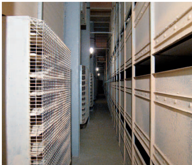
Pressure corridor with a positive pressure of approx 0.1 inches WC
